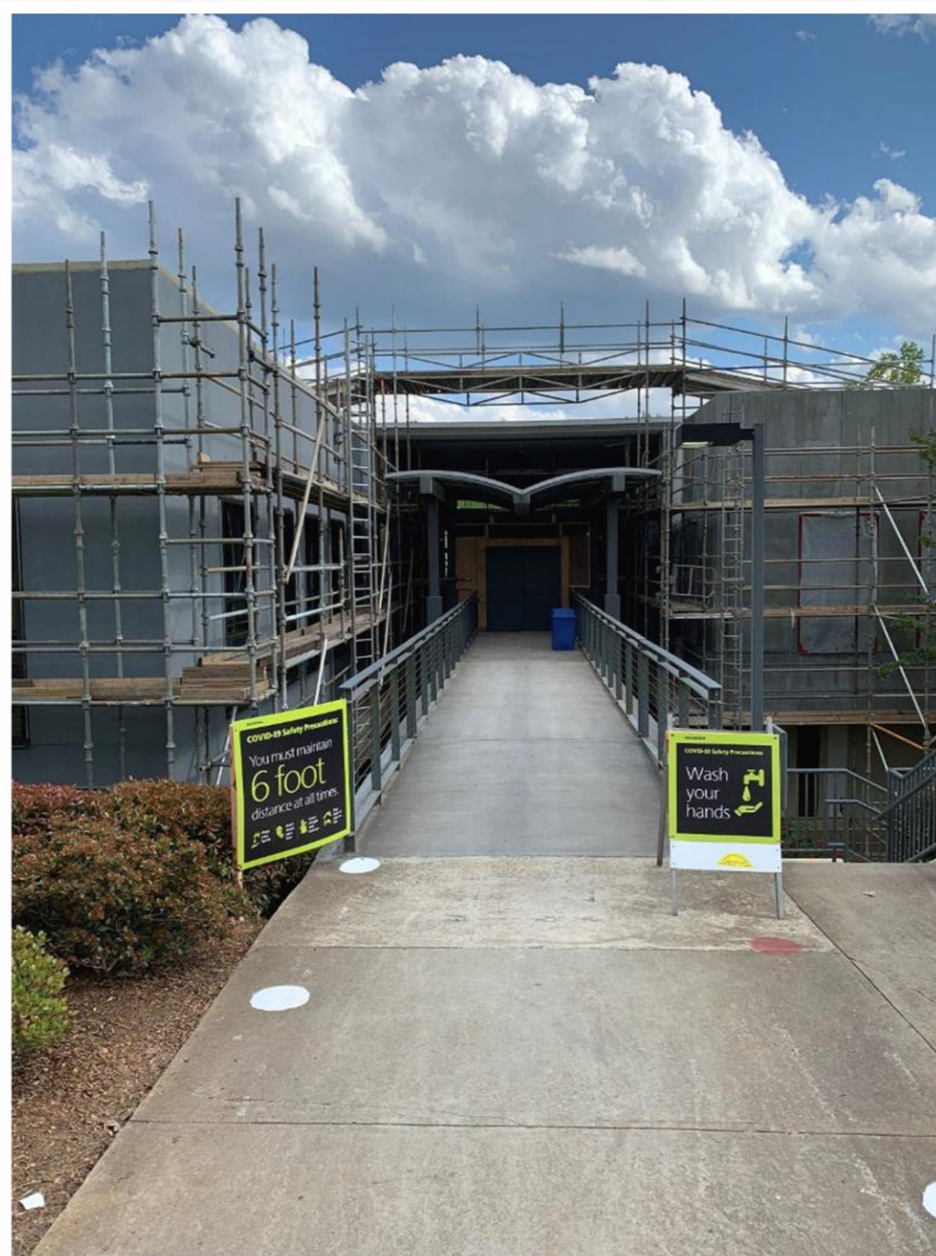
ASHRAE Headquarters during renovation
